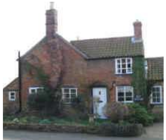
External Chimney at Old Cottage
