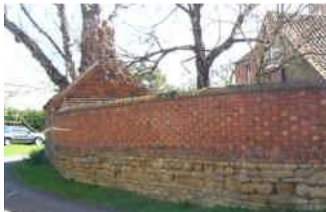
Traditional stone and brick built wall
