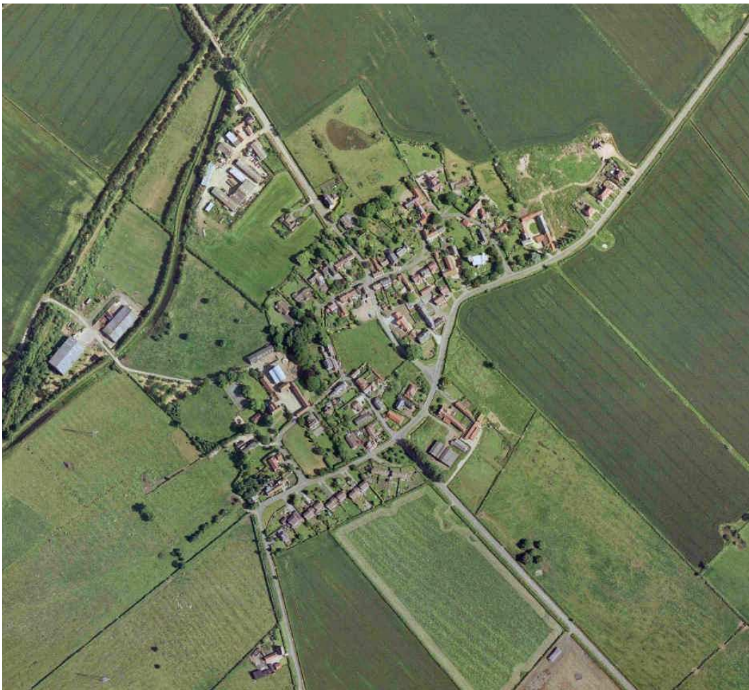
Aerial View of Plungar
